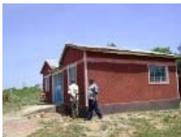
The Completed Barkatado Orphanage Kitchen
